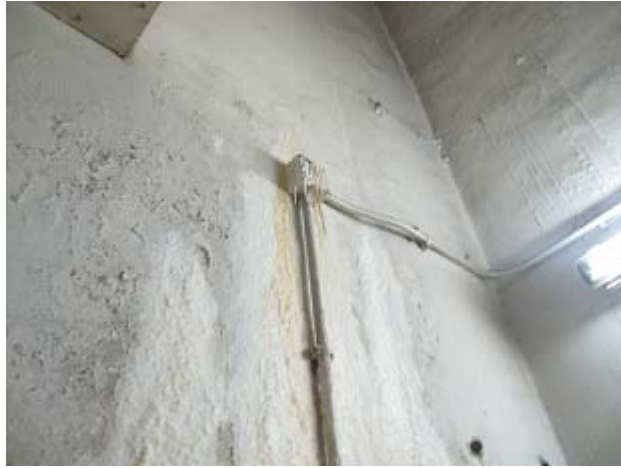
Efflorescence of walls
