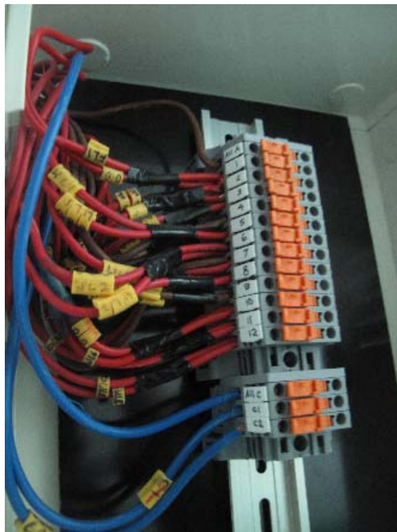
Installation of feeder wires and junction box
