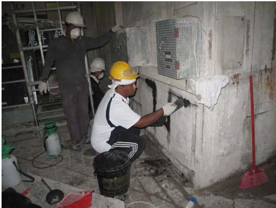
Installation of titanium anode wires and grouting works
