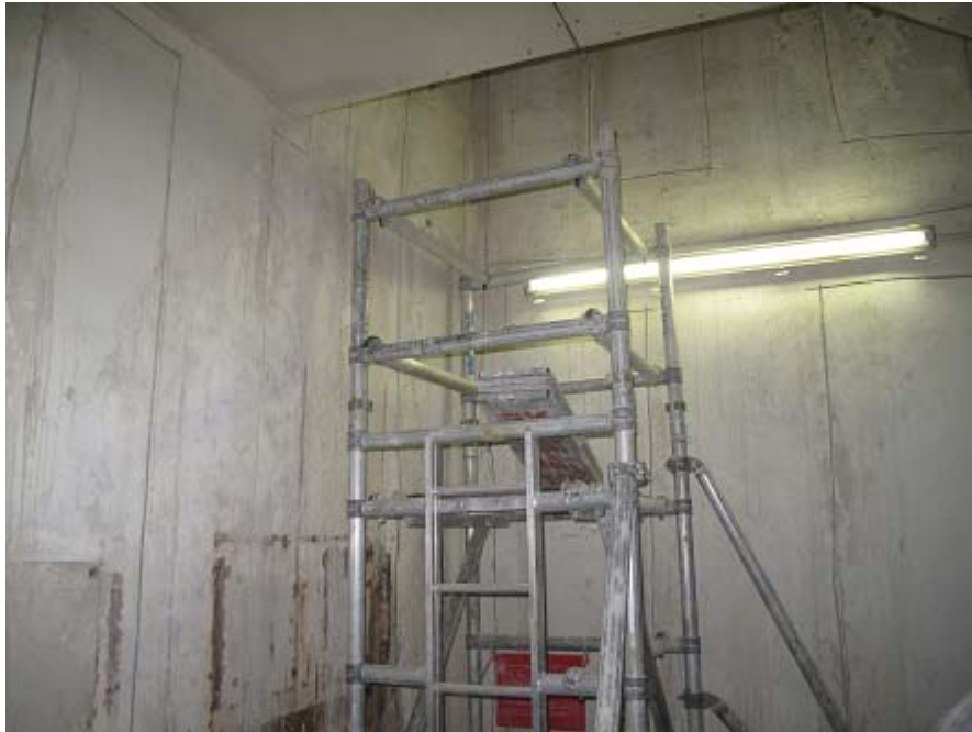
Saw cutting works on walls
