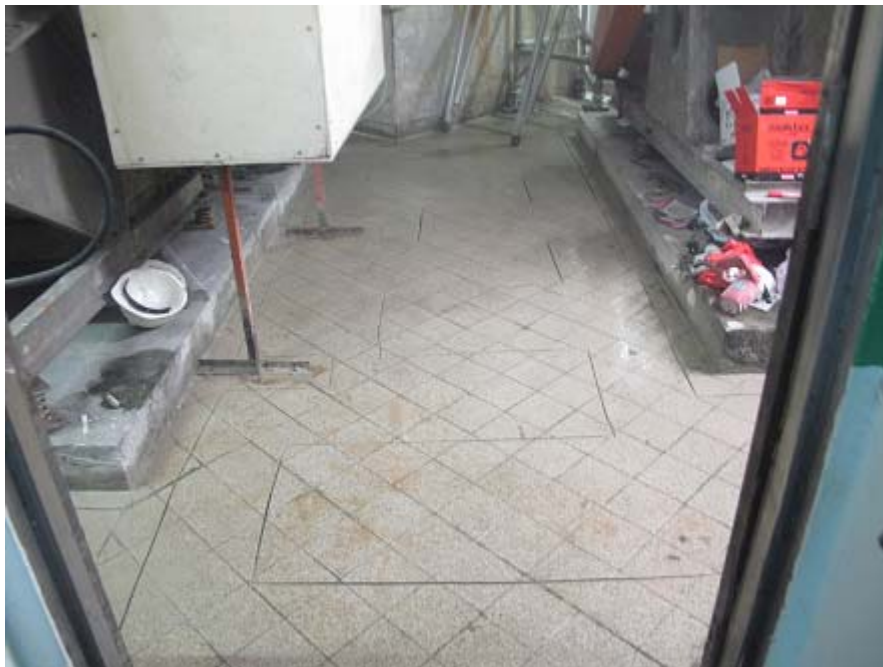
Saw cutting works on floor slab
