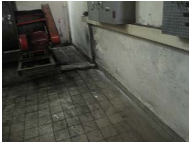
Conditions of existing floor slab
